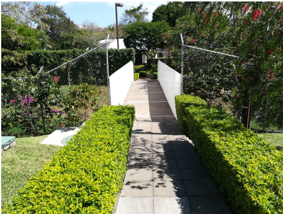
Figura 2.31. Puente 11, Paso peatonal interno Condominio Santa Ana Park
